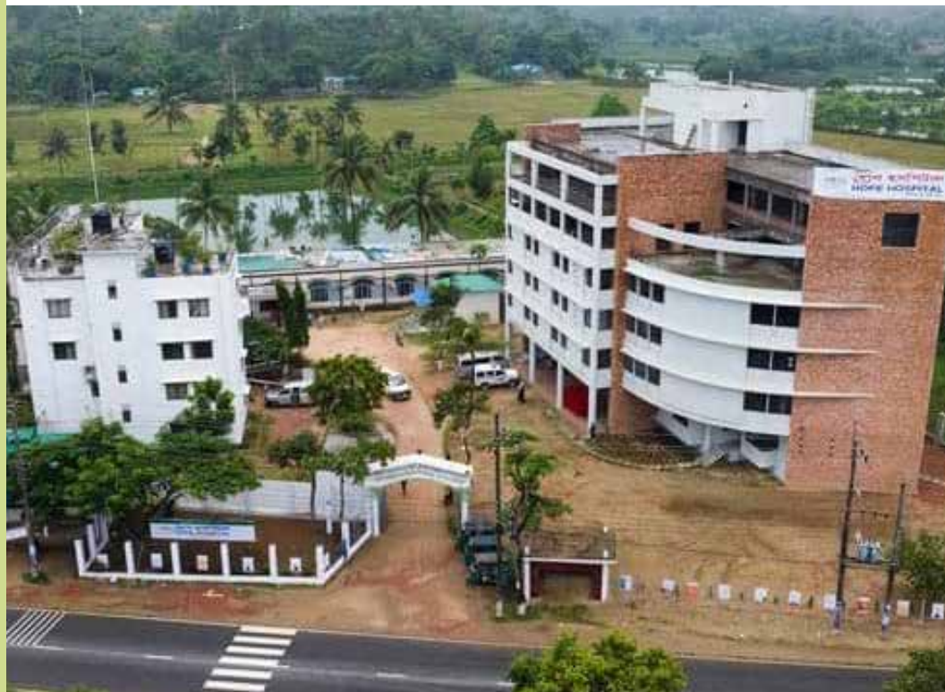
Aerial photography of Hope Foundation Campus in Ramu, taken by Fistula Foundation.
